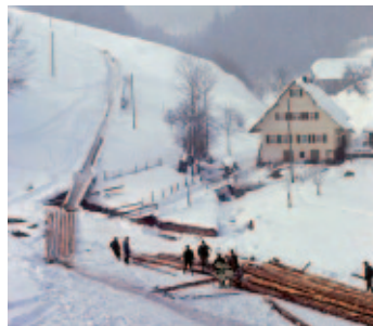
Timber chute in the winter (Bad Rippoldsau / forest around 1950)
