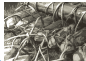
Lashings join logs and raft sections
